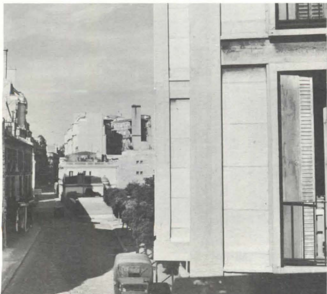
Detail of Perret's apartment house, rue Raynouard, Paris.
