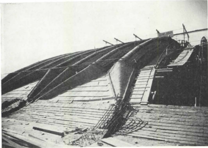
Figure 3—Exposition Palace, Turin, Italy (1947). Prefabricated units (right) of the corrugated roof were consecutively mounted on a tubular scaffolding, fitted together, and joined with poured concrete. Exterior view of roof with elements in place (below). Section of element (below right) is width of one wave, 14\frac{1}{2}' long and slightly more than 1\frac{1}{2}" thick.
