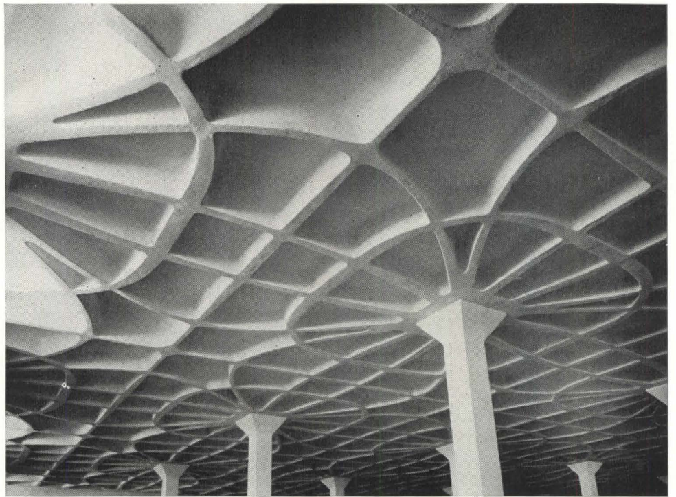
Figure 2—Lanificio Gatti factory, Rome, Italy (1951). Nervi has devised numerous roof systems of precast or poured-in-place, flat-ceiling slabs joined by intricate stiffening networks for distribution of stresses. Ceilings of the Lanificio Gatti factory were poured continuously in place with the forms (above right) set on movable scaffolding. Removal of the scaffolding left a smooth upper surface at floor level and a reticulated ceiling surface underneath, with stiffeners collecting the load at column heads (above and right).
