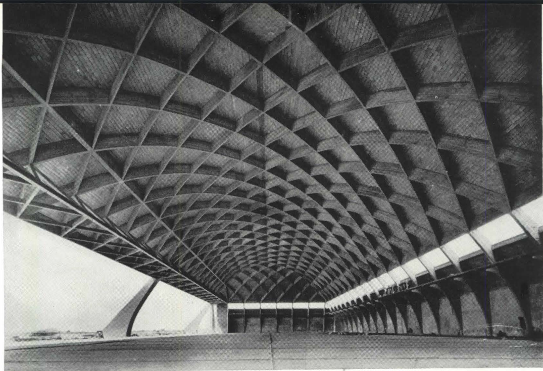
Figure 1—airplane hangar near Rome, Italy (1938).
