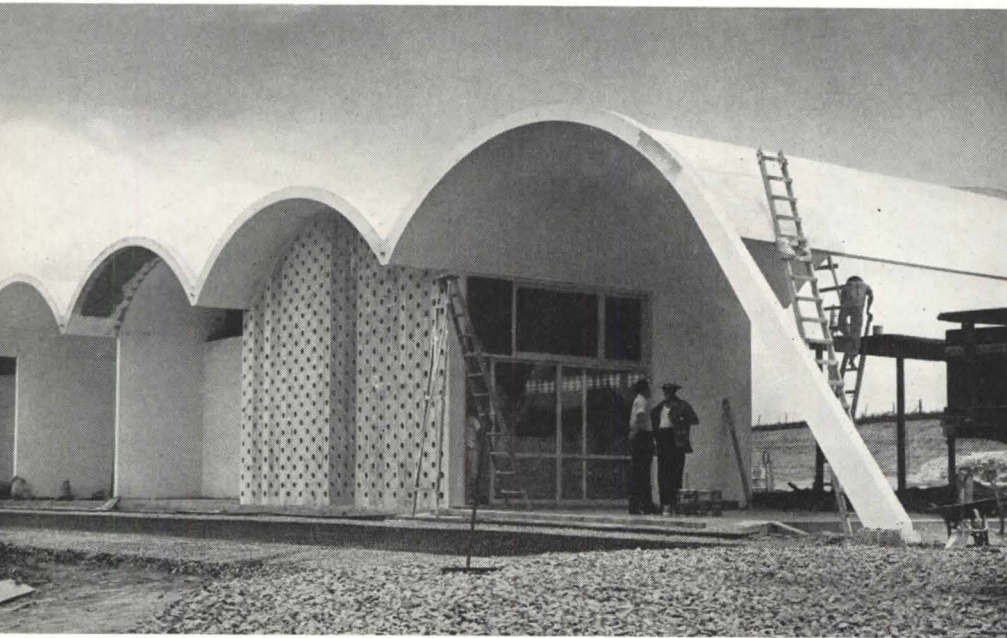
Club dos 500, São Paulo (an automobile service station). "Customer-attraction" pylon (above); details of repetitive barrel-vaults over administrative area (left and below); two views of service area (acrosspage). Elements of the plan are: (1) portico; (2) office; (3) rest rooms; (4) offices; (5) storage; (6) pumps; (7) lubrication pits.
