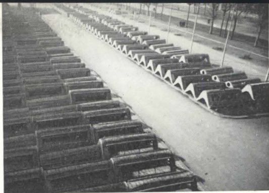
Figure 3—Exposition Palace, Turin, Italy (1947). Prefabricated units (right) of the corrugated roof were consecutively mounted on a tubular scaffolding, fitted together, and joined with poured concrete. Exterior view of roof with elements in place (below). Section of element (below right) is width of one wave, 14\frac{1}{2}' long and slightly more than 1\frac{1}{2}" thick.
