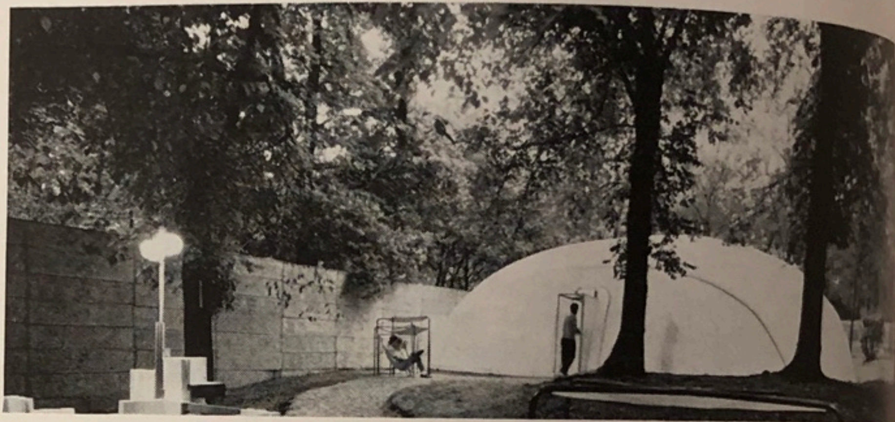
→ Inflatable plastic dome made by Plasteco Milano is translucent.
