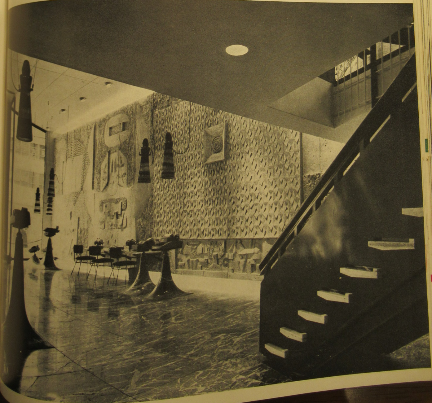
Below: Heavy steel reinforcement demanded by the building department thickens the stairs in profile view. Marble treads, supposed to have been lightly suspended in the sides have been unnecessarily reinforced with steel plates underneath.
