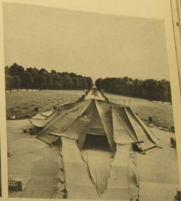
Partition for fashion shows and concerts spreads out below the steps of the Stupinigt palace in Turin. Draped in violet-purple, with a scarlet lining showing through at the folds, the elegant structure holds its own against the baroque composition of the little jewel of a palace. The structure is put together of standard steel tubing by means of adjustable joints. The tubes are painted yellow and orange, with black leg posts. The metal furniture inside is lacquered blue, the canvas rug natural. There is room inside 111-foot diameter for stage, bar, orchestra, runway.
