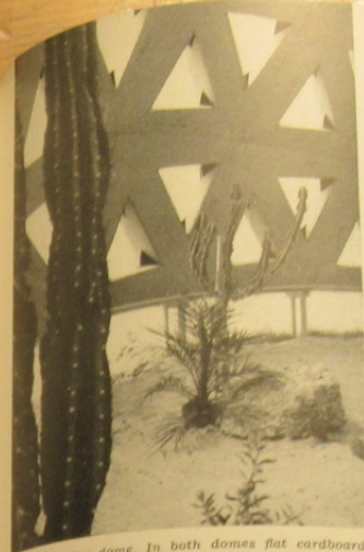
Cactus display dome. In both domes flat cardboard components were folded into 3-dimensional triangles, stapled into groups, then the groups into a dome.
