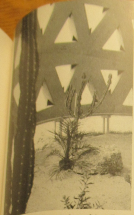
...display dome. In both domes flat cardboard components were folded into 3-dimensional triangles, grouped into groups, then the groups into a dome.
