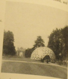
Cactus display dome. In both domes flat cardboard components were folded into 3-dimensional triangles, stapled into groups, then the groups into a dome.
