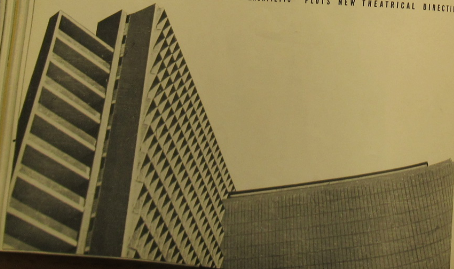
Hotel annex, from southwest
