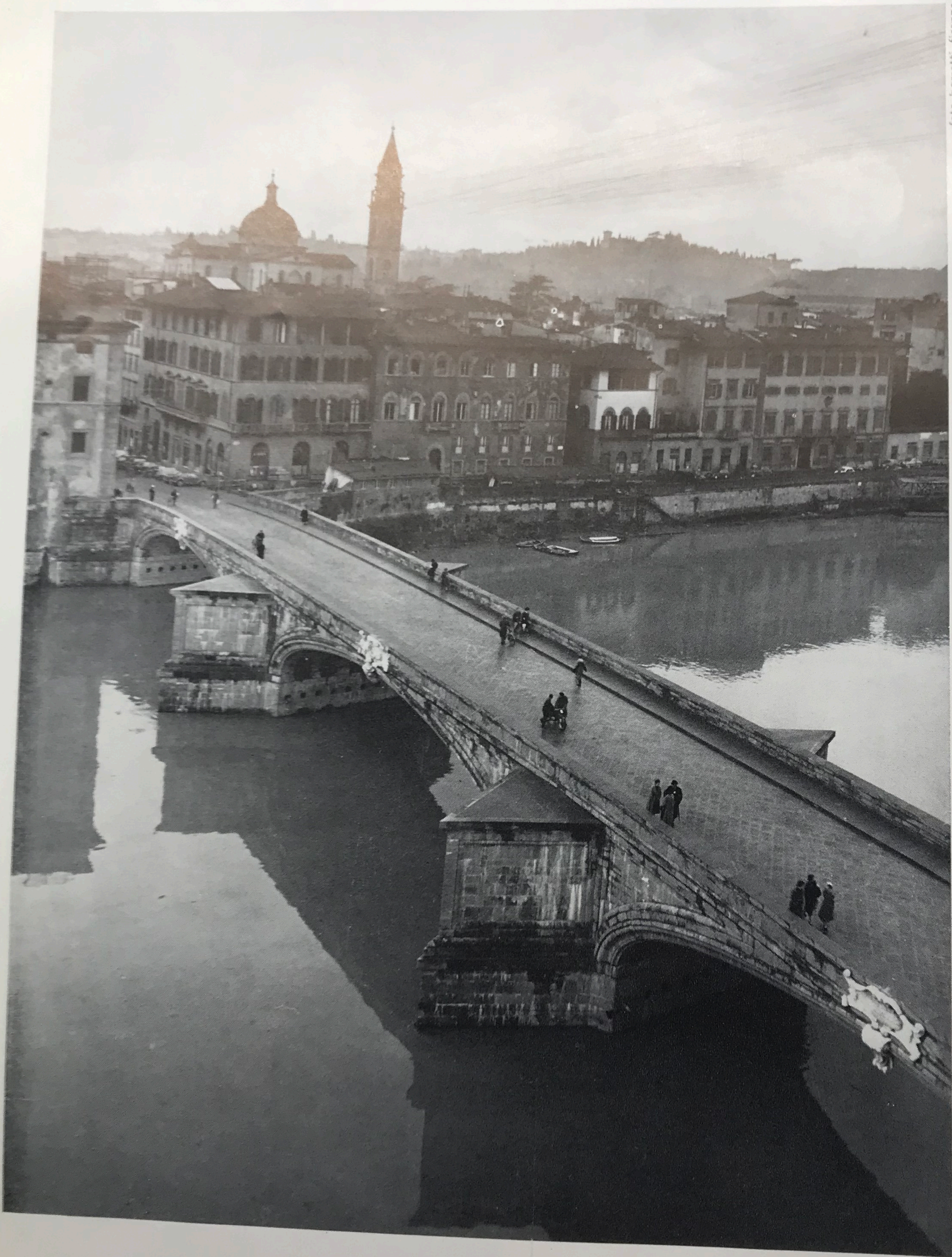
Challenging modern engineering theories, Ponte a Santa Trinita was restored with its original delicate, shallow arches, proven adequate for any load.
