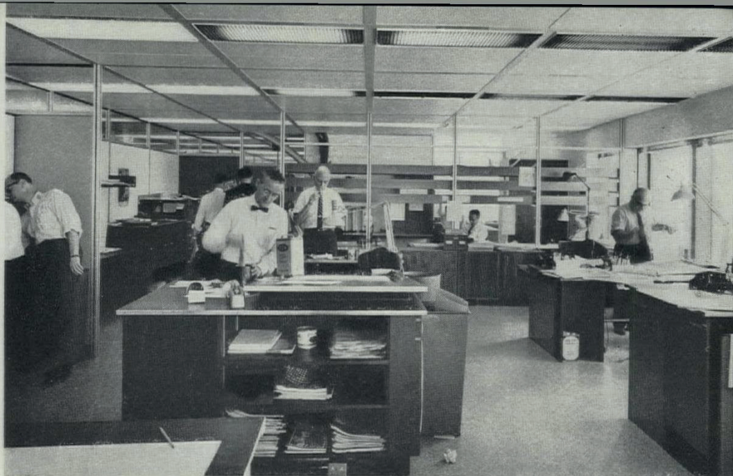
In LIFE's layout room partition posts on grid intersections support only space-dividing shelves.
