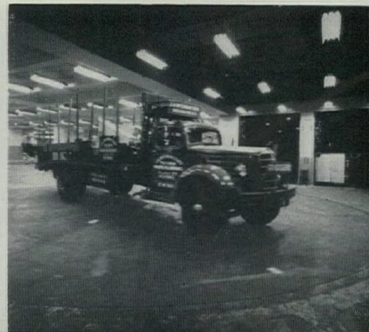
... and the truck turntable in the subbasement.
