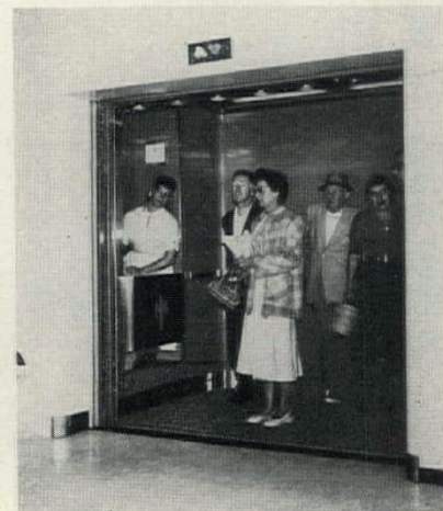
5. Elevator has operator's booth.
