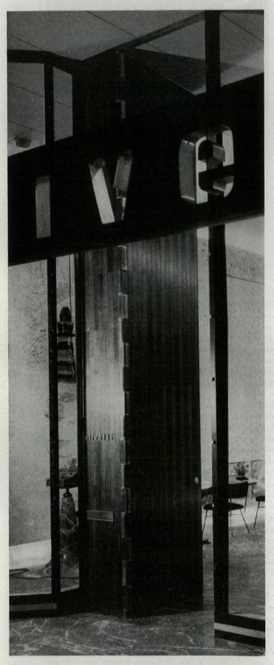
The great door,  $16' \times 3' \cdot 5''$ , of matched walnut sections, has continuous brass hinge, can easily be hand operated, but is hard to keep quietly lubricated in New York's damp summer weather.
