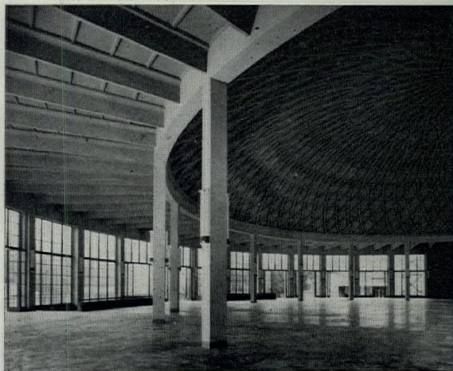
The web of strips visible in the ceiling does not support the cupola. That job is done by curved diamond shaped slabs which rest between and above the ribs (which are only separators and stiffeners).
