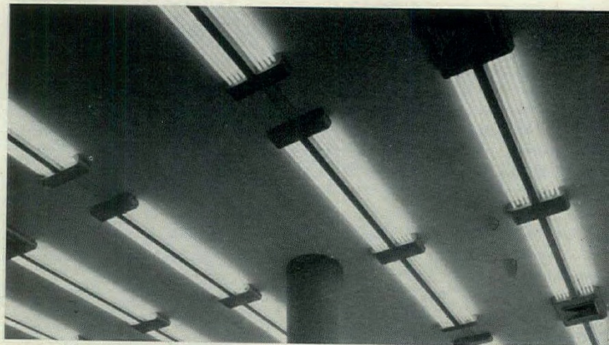
DUCT SYSTEM PERMITS LIGHTING FIXTURES OR LAMPS TO RUN PARALLEL TO DUCTS (ABOVE) OR AT RIGHT ANGLES (BELOW), SPACED AT ANY INTERVALS
