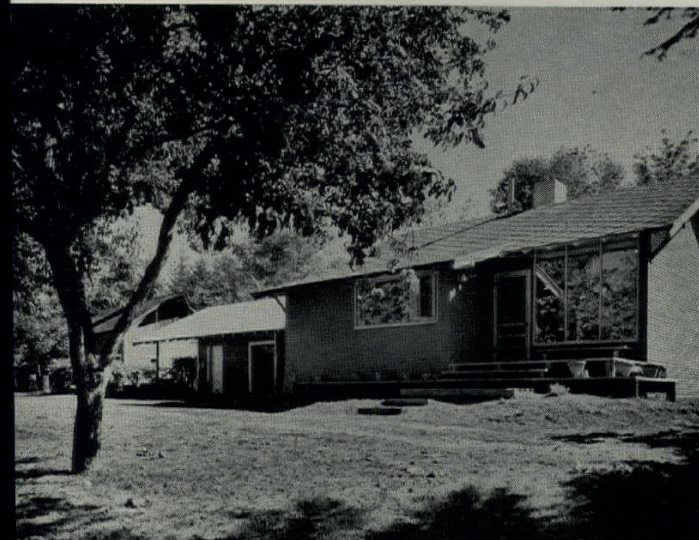
OLD PORCHES WERE REMOVED, NEW ENTRANCE SUBSTITUTED
