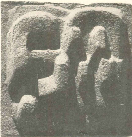
The use of sculptured inserts to provide shadow interest for a building façade is shown in this study for a school soon to be built. Each insert would be individually designed. A typical one is shown above
