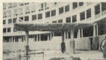
Top: Conference-Assembly building has folded walls to support its folded roof at the ends. Both show visually in the Main Assembly room. One section of a side wall has staggered concrete framing, serving both as structure and fenestration, giving a playful contrast to the more monumental end wall. Left and below: Large canopy to Secretariat is two abutting conoids; small one is flat, ribbed slab
